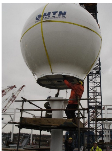
Installing the satellite system
